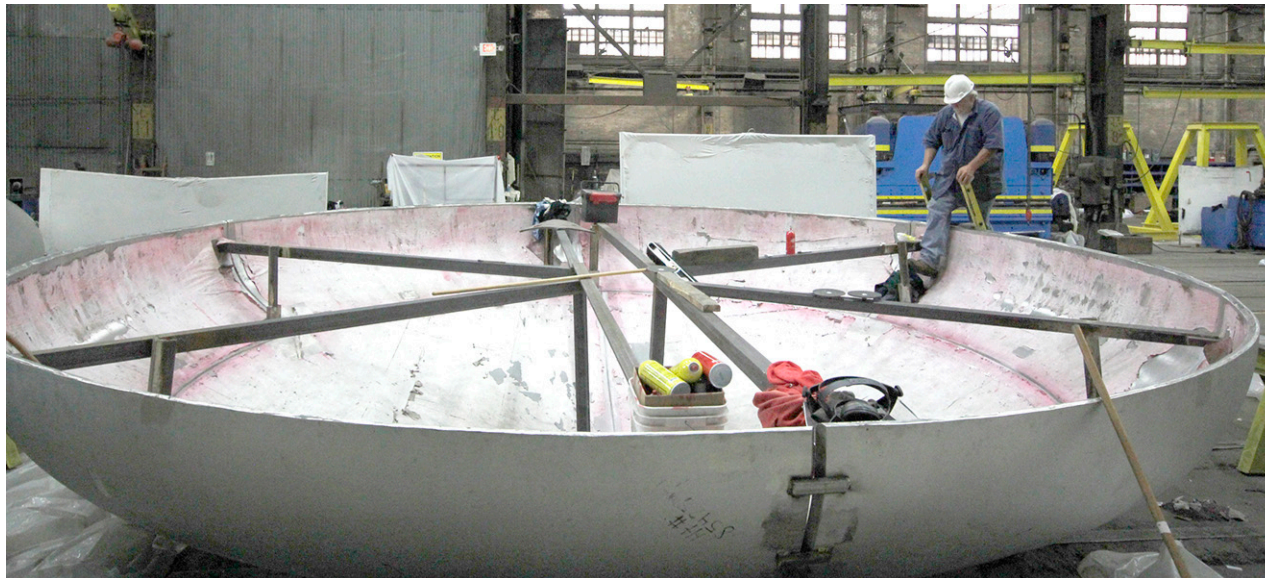
Drain tank head positioned for welding at Joseph Oat Corp. in Camden, NJ Photo: US ITER
